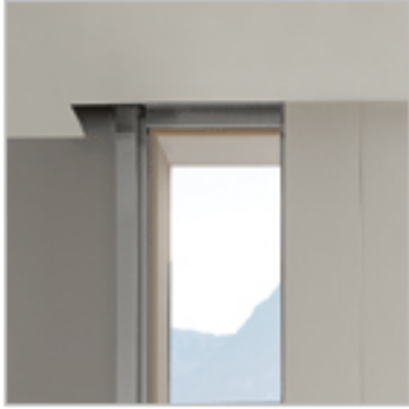
Line flush with the ceiling
